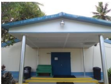
Figure 3: The roof after the repairs
