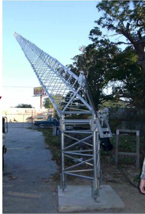
Folding over a 72 ft. tower (model rated at over 34 sq. ft. at 80 mph wind speed.)
